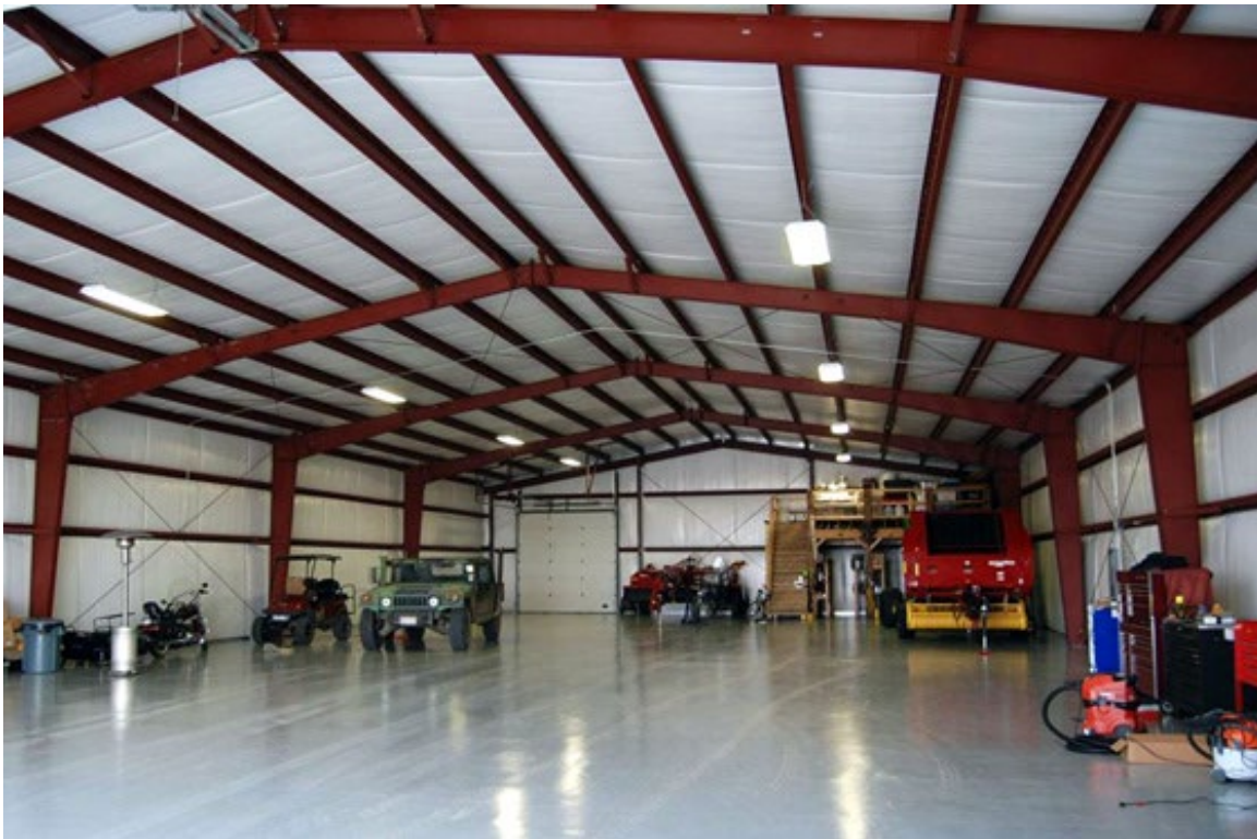
Figure 14. Interior of the pre-engineered steel building.
