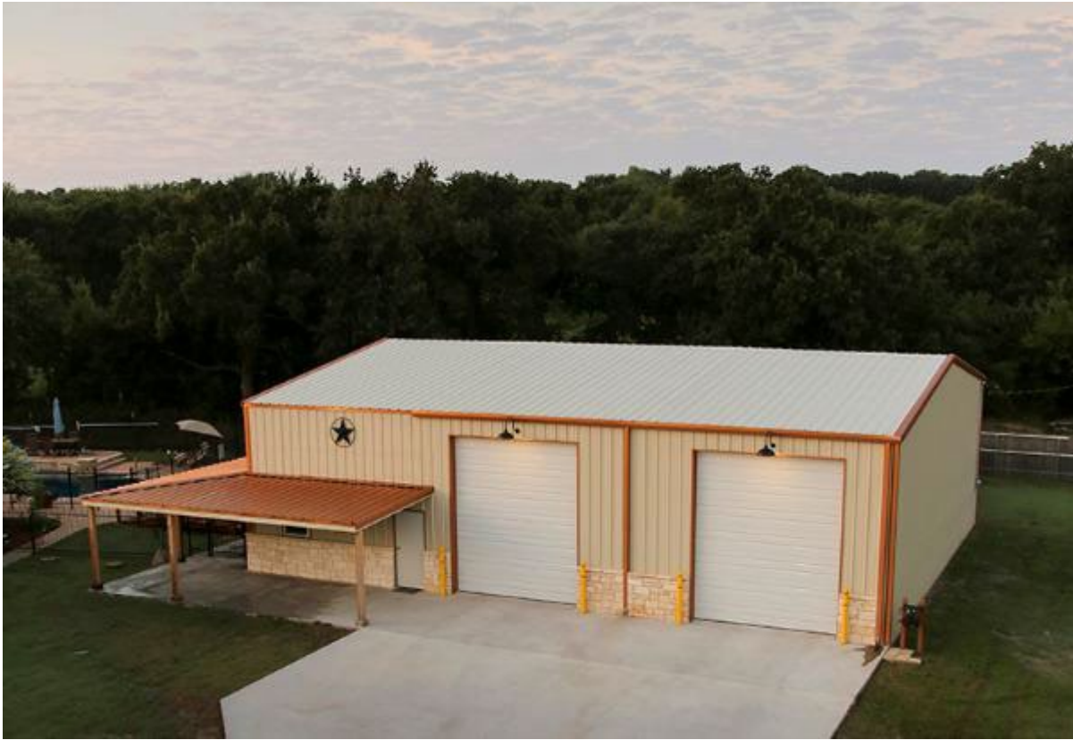
Figure 13. Exterior of the pre-engineered steel building.
