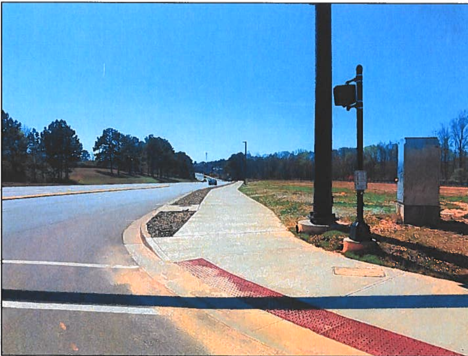
A new sidepath along an arterial street
